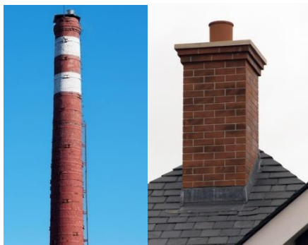
Figura 8. Chimeneas Fuentes: industrialaccess.com y www.wessexbps.co.uk, 2018
