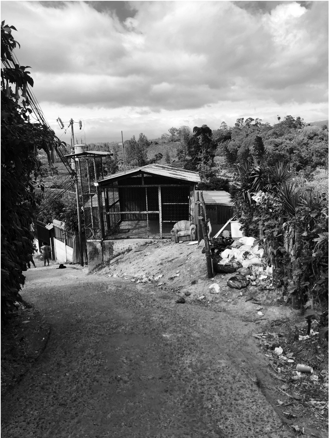
AyA Repumping Station of Calle Los Mangos
