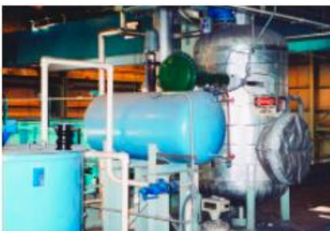
Figura 5.7 Separador flash Eclipse® Model 706, de la marca MAGNETROL (Tomado de magnetrol.com/en/industries-applications/power-generation/flash-tanks )
