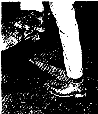
Routine maintenance activities can cause disturbance of ACM if workers are not properly trained in operations and maintenance procedures. Here, a worker carelessly contacts ACM, possibly damaging it.
